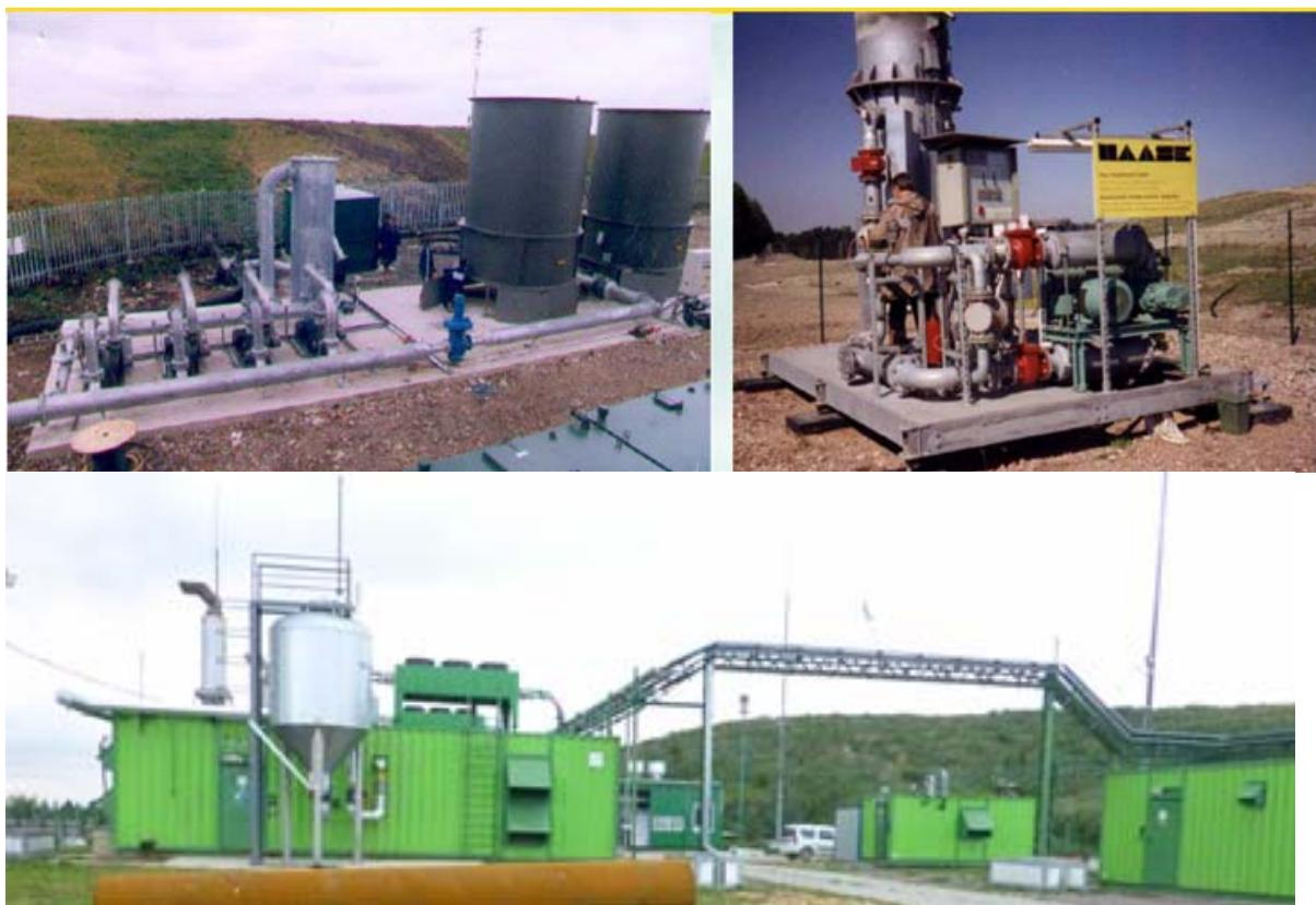
Figure 7 – Booster and flares system (top) booster and CHP units (above)
