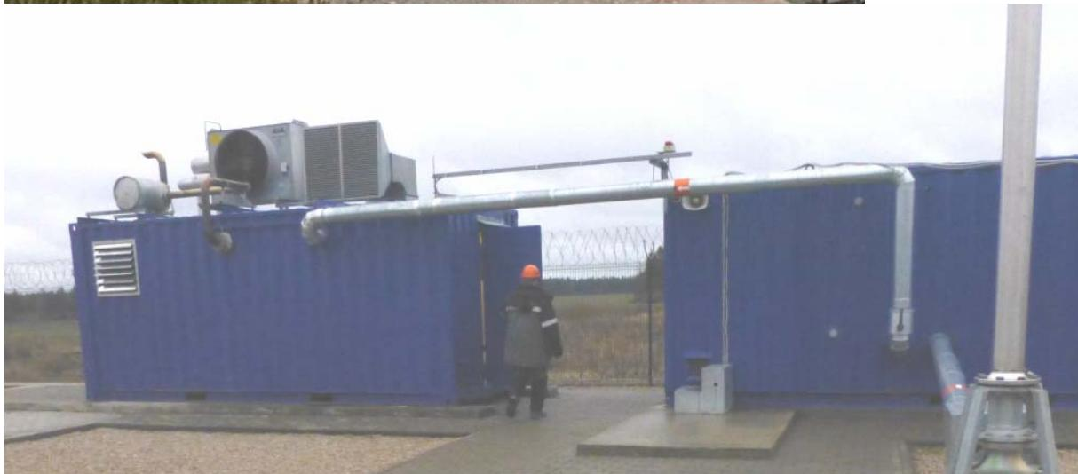
Figure 8 Containerised booster system and gensets (CHP units) Clarke Energy Ltd. in Wales (top) and Vireo in Belarus (below)
